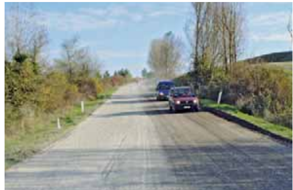
Recycled lane can be used after compaction.
