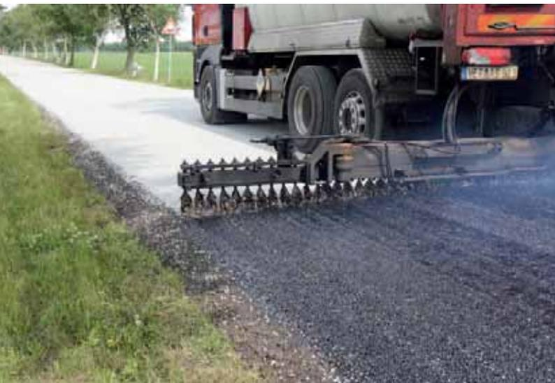
Spraying hot bitumen for the surface layer.
