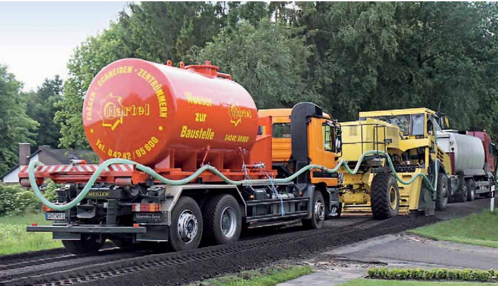
BOMAG MPH 125 milling recycler mixing foamed bitumen and water.
