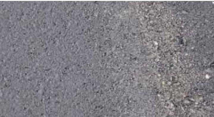
Fig.14: Quality aspect: Smooth longitudinal joints after horizontal directed compaction.
