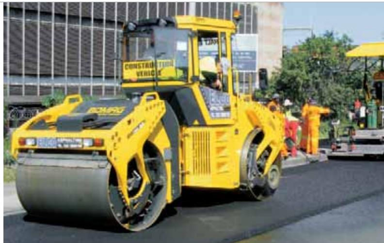
Fig. 6: In the „hot zone“: BW 151 AD-AM in operation.
