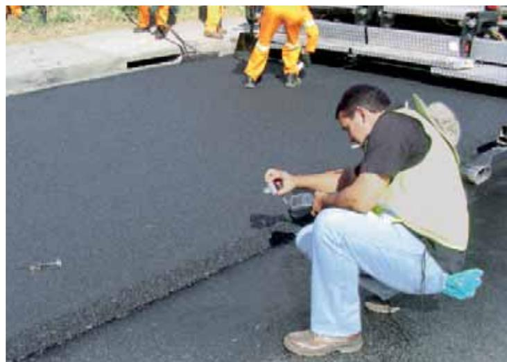
Fig. 7: Continuous temperature control at site.
