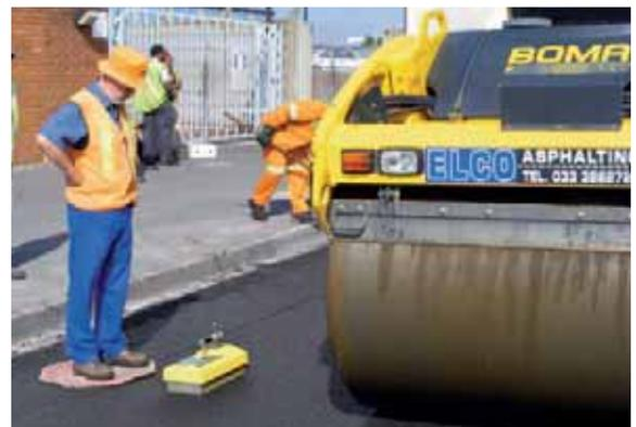
Fig.13: Calibration to density with a nuclear gauge.
