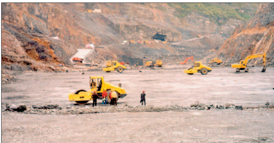
Compaction of 1000 mm rockfill layers of lower dam body.
