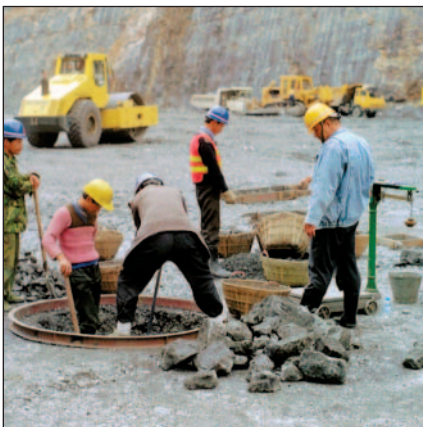
Rockfill grading and density control.
