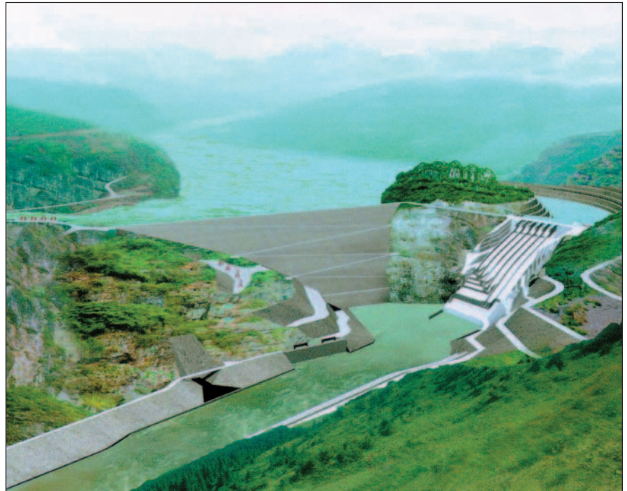
Shuibuya rockfill dam and hydro power plant.
