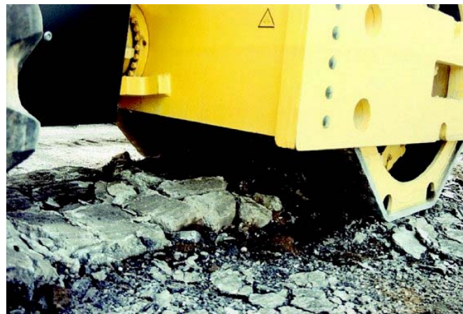
Fig. 12: De-tensioning of the concrete superstructure on the A9 motorway at the Schkeuditzer Kreuz
