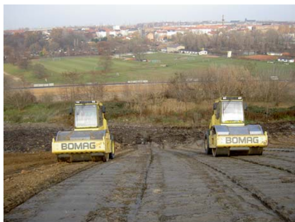
Fig. 14: The wash-board pattern ensures good bonding between the individual layers
