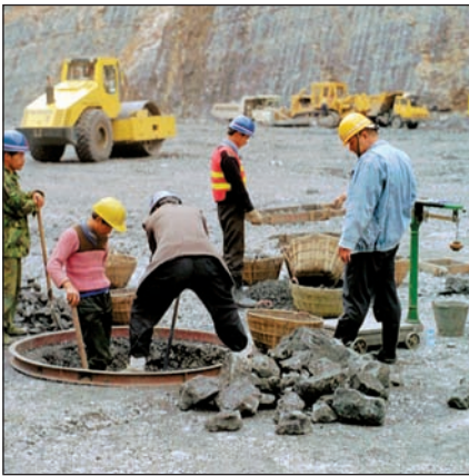
Rockfill grading and density control.
