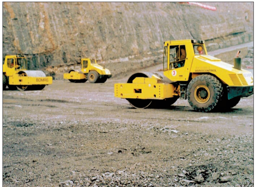
25 t VARIOCONTROL roller in automatic mode on a 1000 mm rockfill layer.
