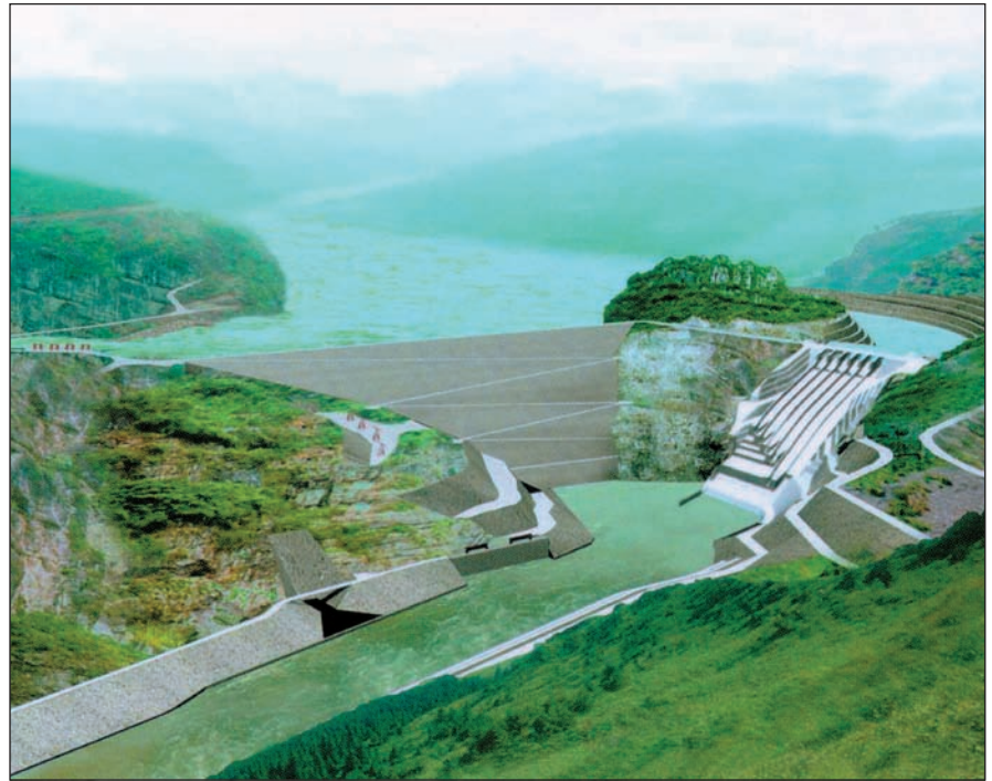
Shuibuya rockfill dam and hydro power plant.
